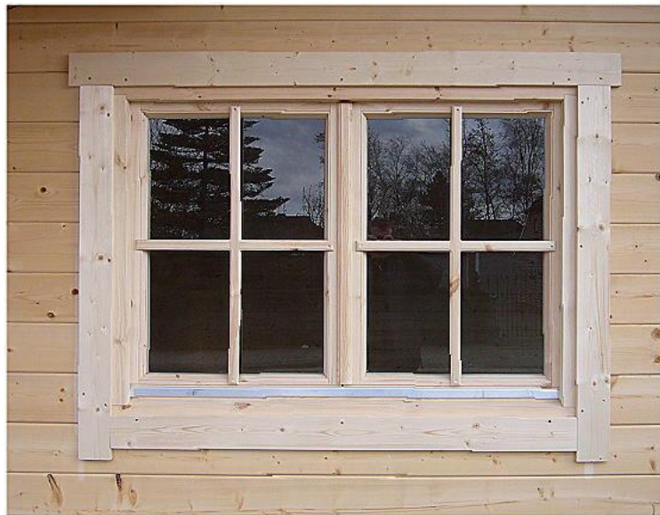
Picture 9: Door and window frame for logs smaller than 70 mm, after production 7/2007 (t-bar)
